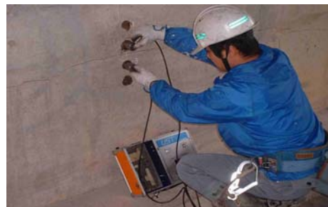
●超音波測定 (ひび割れ深さ)
